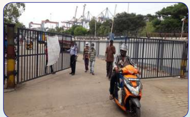
Newly constructed gate at Vizag FH to restrict unauthorized entry
