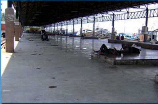
Improved condition of Thopumpady fisheries harbour
