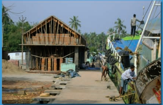
Rennovation works going on at Valappattanam harbour
